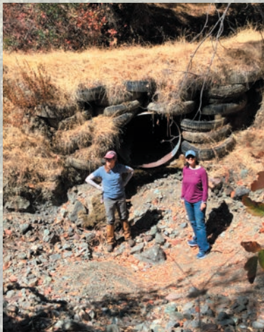
ACR staff on site shows the human scale of a culvert reinforced by truck and tractor tires, installed when the Modini property was a commercial cattle ranch.
