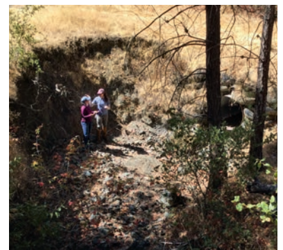
The human scale of the steep head cut to the left of the culvert outflow, where storm water has carved an abrupt vertical drop causing sediment to flow into the stream.
