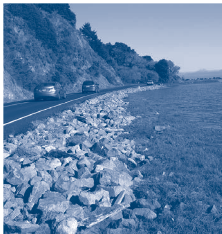
Figure 3. Shoreline Highway was recently armored with a rock surface to reduce tidal erosion and flooding on the east side of Bolinas Lagoon.
